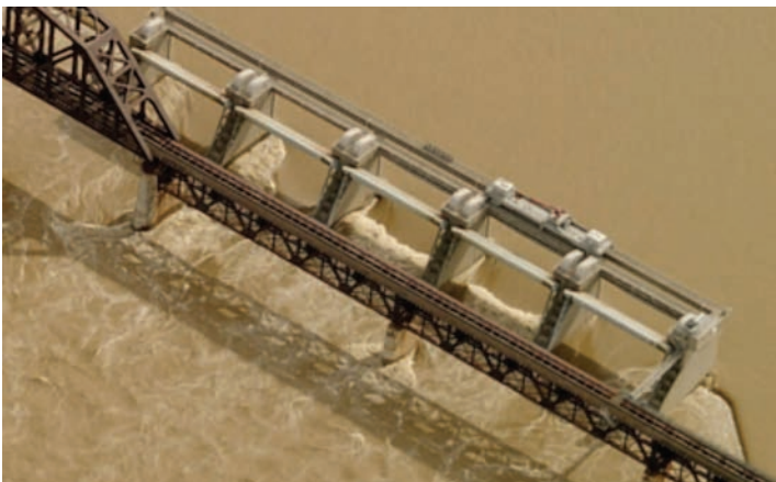
Figure 4 -McAlpine Lock and Dam upper gates 5
